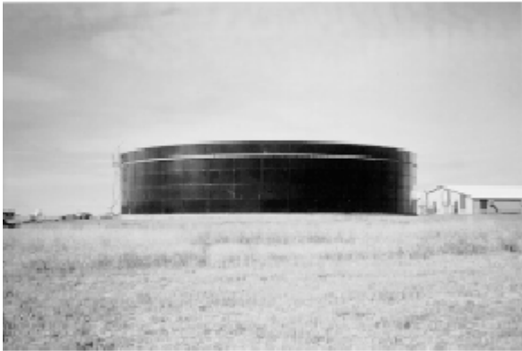
Figure 10. Above ground concrete liquid manure storage that can be used in places where soil conditions would pose risk to drinking water if earthen storages were used. (Source: PAMI, 1997b).
