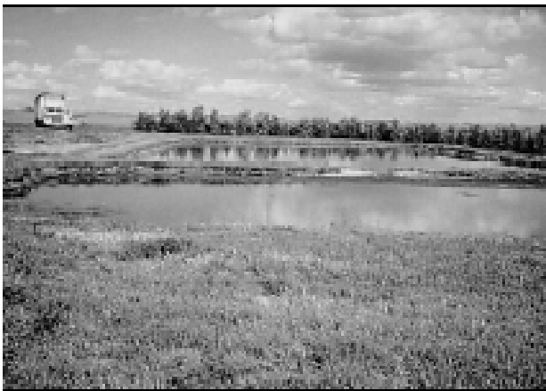
Figure 12. Earthen manure storage (SAF, 1997).
